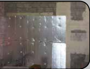
Interior walls on concrete block
