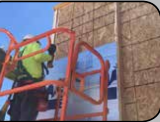
Behind cladding over wood stud walls
