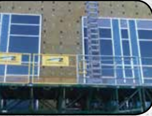
Behind cladding over steel stud walls
